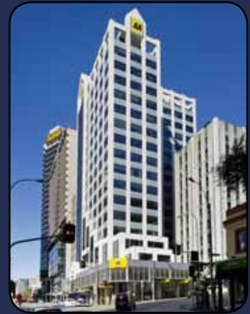
AA Centre 99 Albert Street, Auckland
