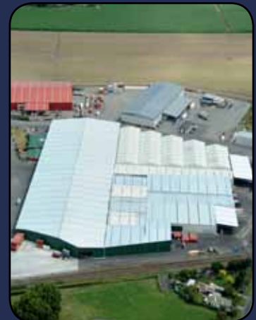
Heinz Wattie's National Distribution Centre 113 Elwood Road, Tomoana, Hastings
